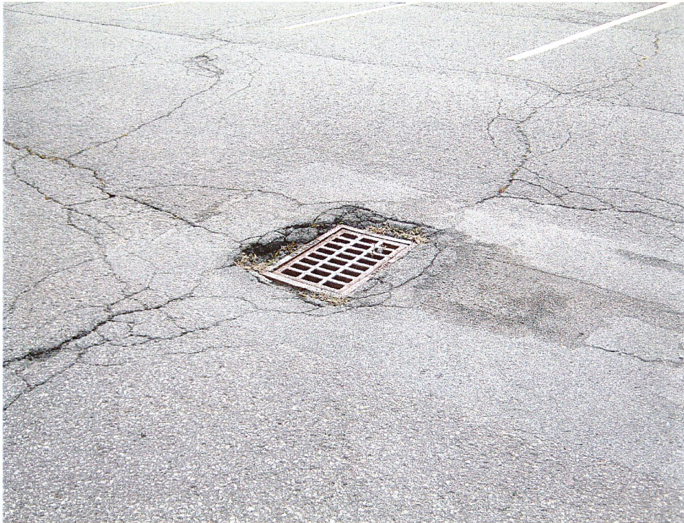
Photo 7: View of a surface water catch basin located within the Site property.
