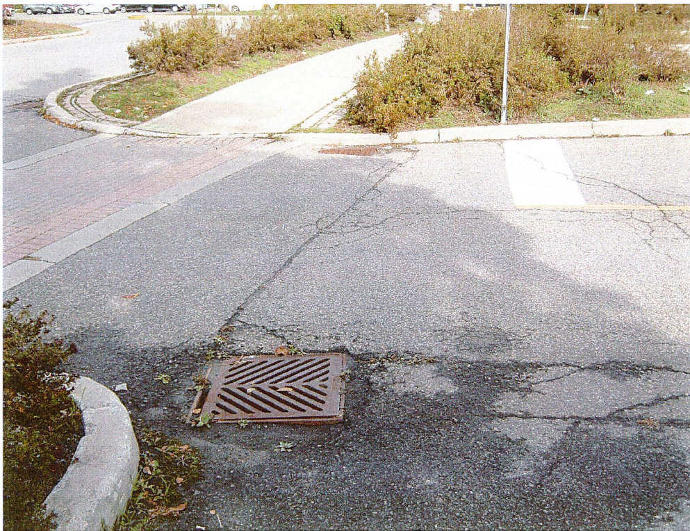
Photo 2: View facing north of 2 surface water catch basins located at the entrance onto the Site property off Lancelot Drive.
