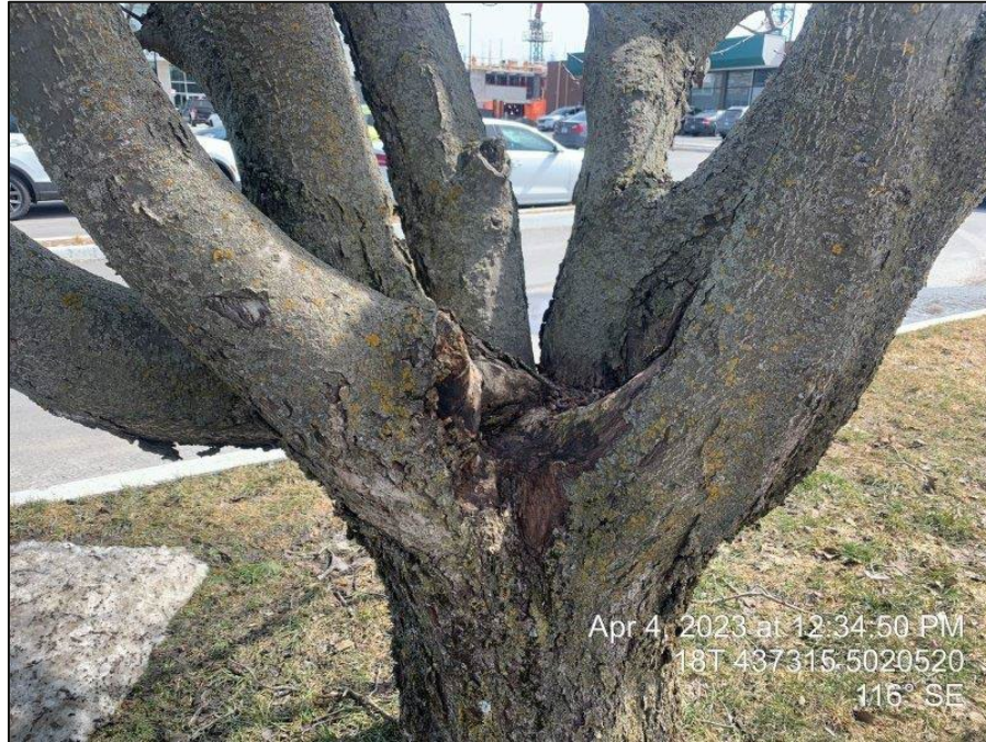
Photo 1: View of the crotch decay and poor structure of Tree #14 – Oakleaf Mountain Ash
