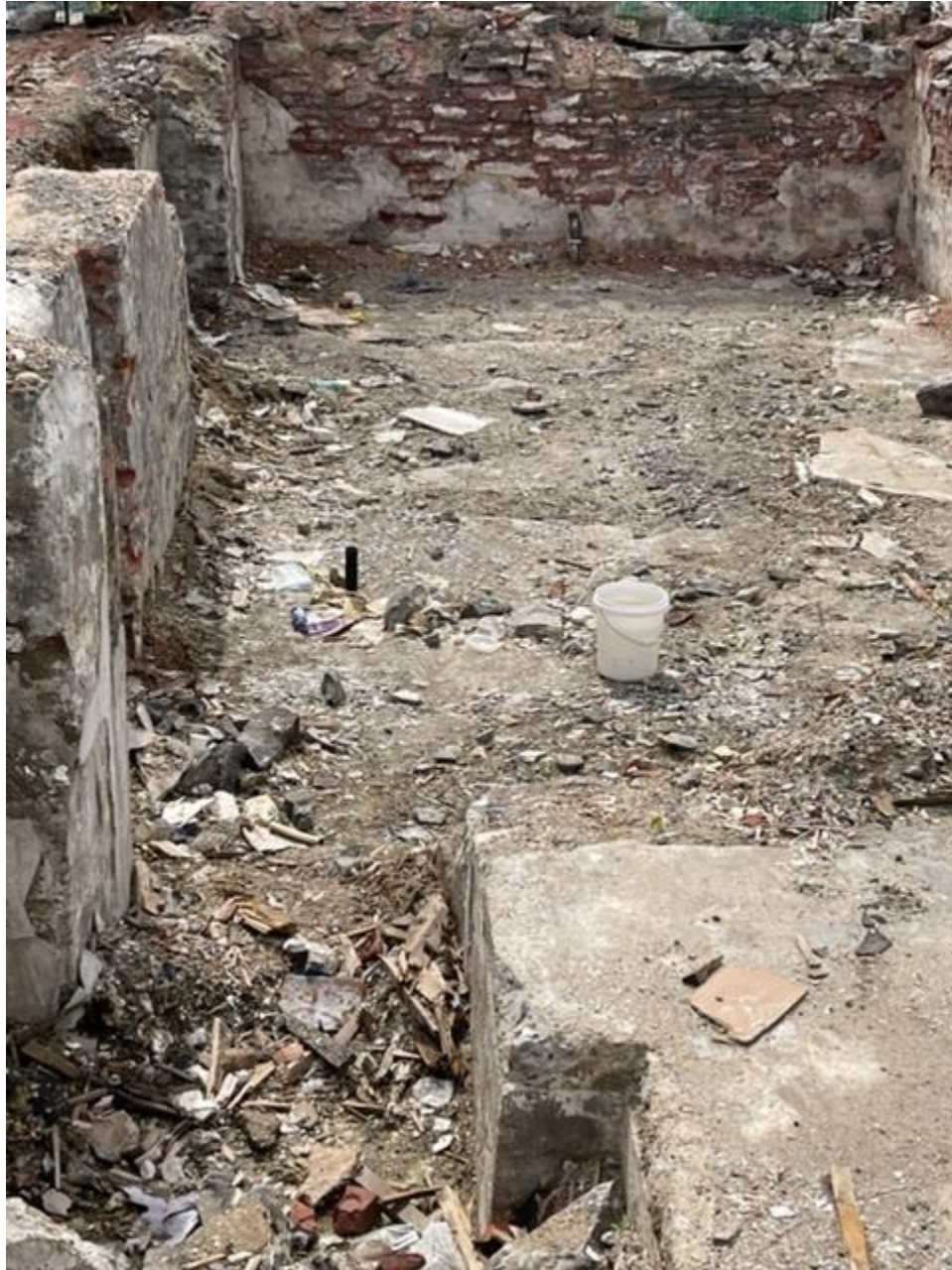
Image 3 - EXMW2 within the basement foundation
