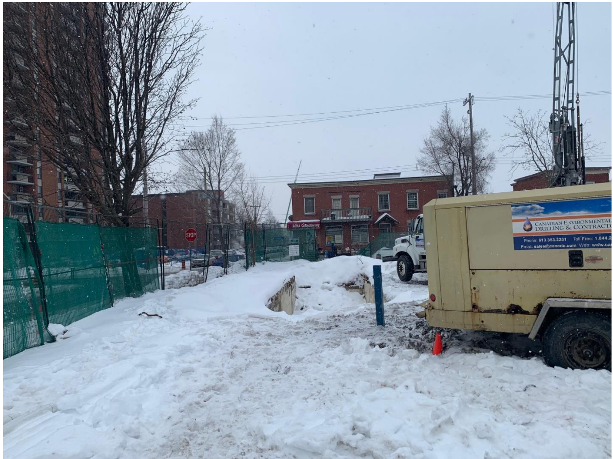
Image 1 – Monitoring Well 4, facing west (later decommissioned)
