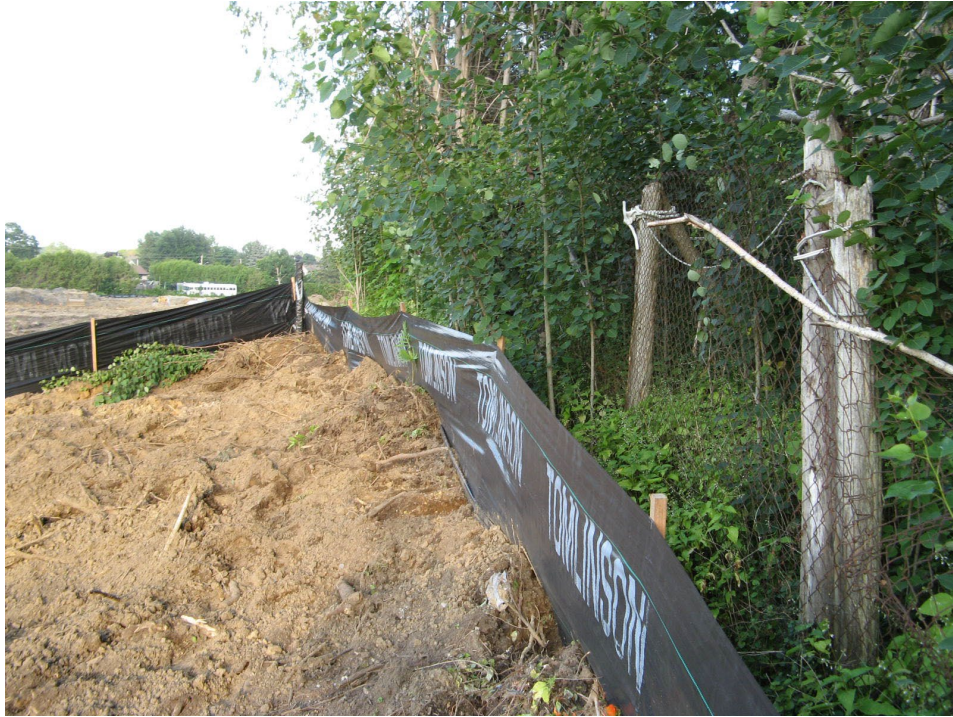
Photo 5 – Typical initial regrading and silt fencing adjacent to the rear (north) of 2993 and 2997 Navan Road. View looking east
