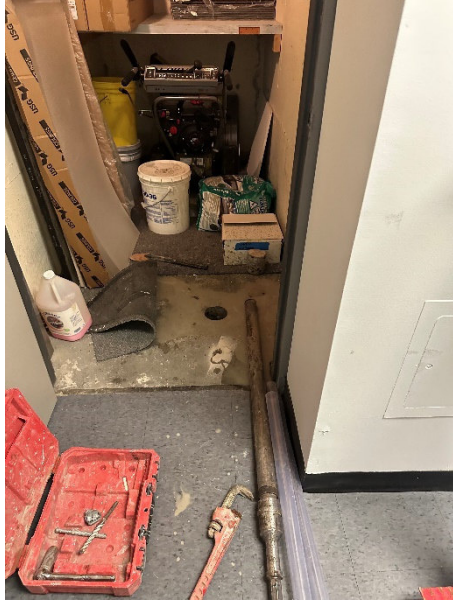
Location of Borehole BH1
