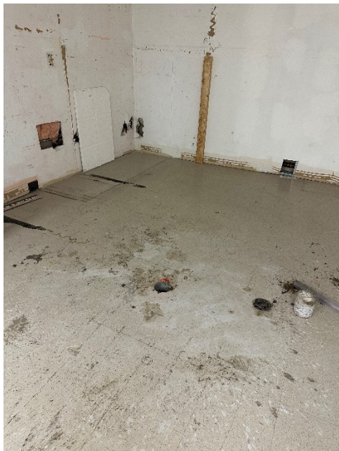
Location of Borehole BH3
