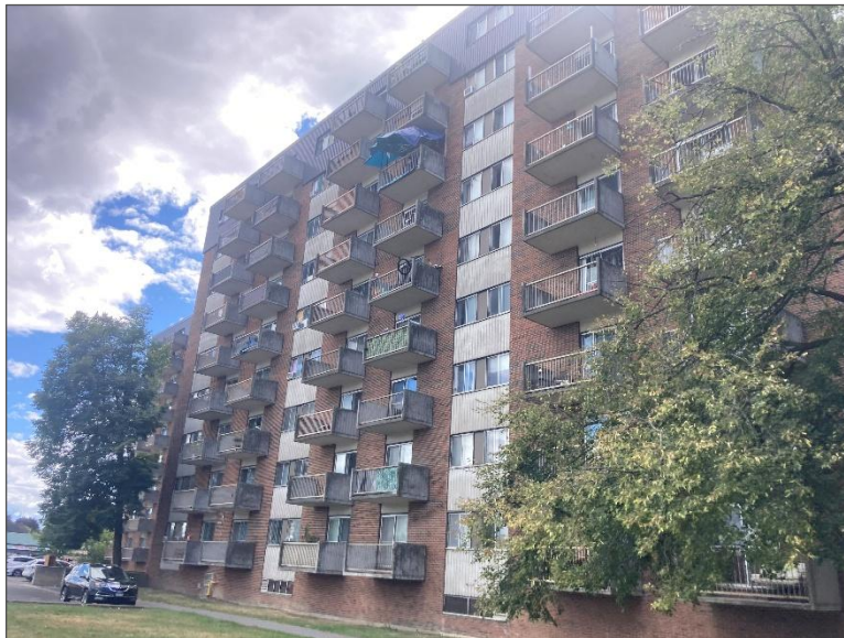
Photo 2 – Site Building B (east elevation).
