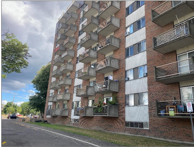
Photo 1 – Site Building A (north elevation).
