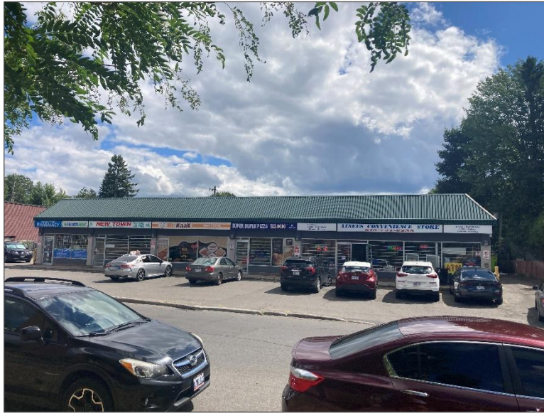
Photo 7 – Property located south of the Site.
