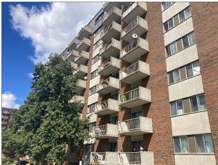
Photo 4 – Site Building B (west elevation).
