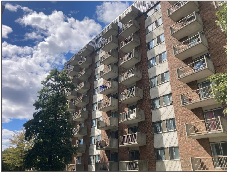
Photo 3 – Site Building A (south elevation).
