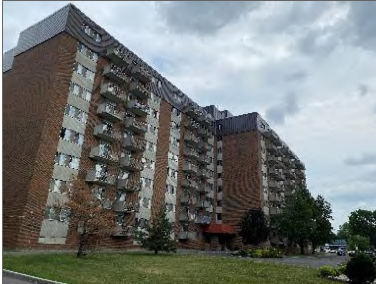
Photo 5 – Site Building B (west elevation).
