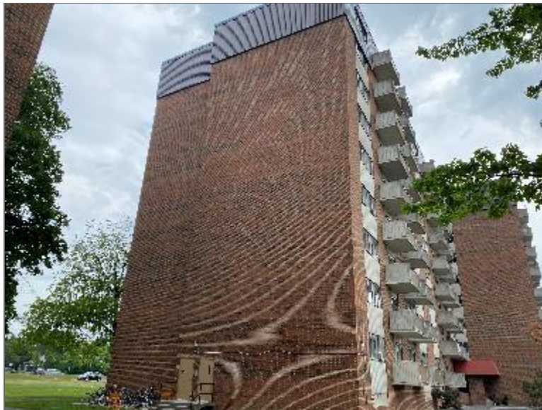
Photo 4 – Site Building B (north elevation).
