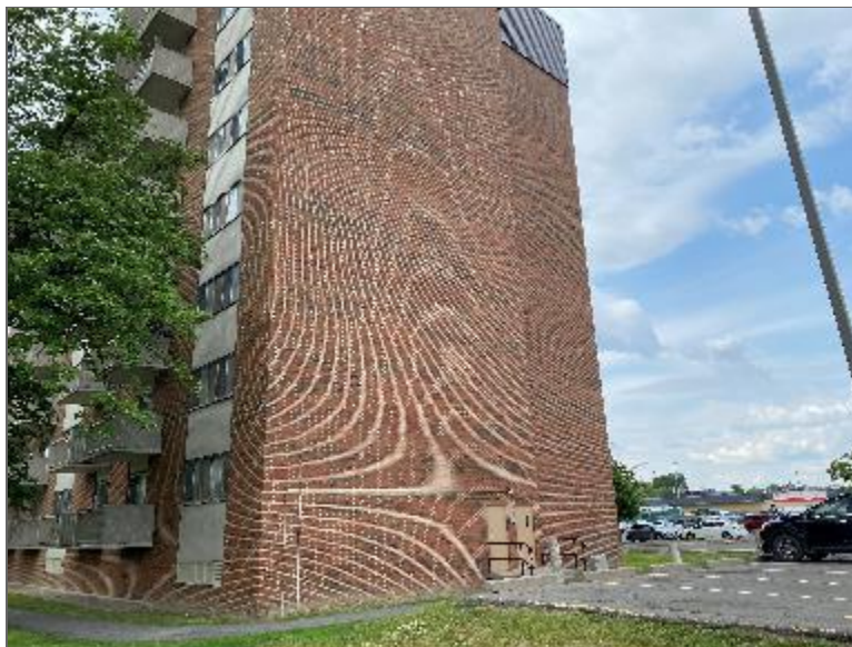
Photo 2 – Site Building A (east elevation).
