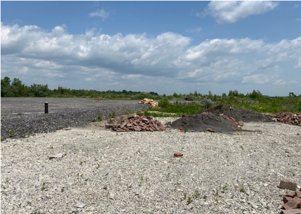
Photograph 1: View looking east, from the south side of the subject site.
