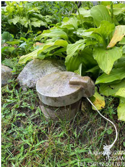
Photo 8 - Observation well at 4885 Hawthorne Road used during pumping test for monitoring of potential interference effects.
