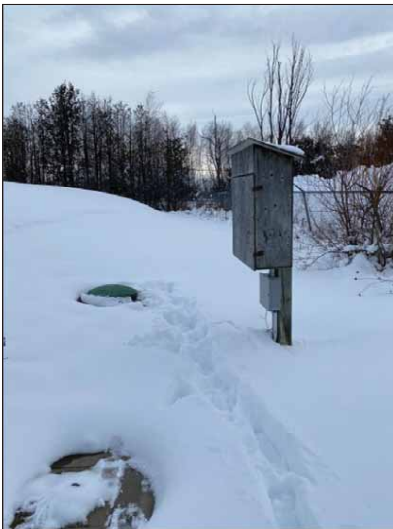
Photograph 5: View of access hatches and electrical systems associated with the septic system located on the south property boundary.
