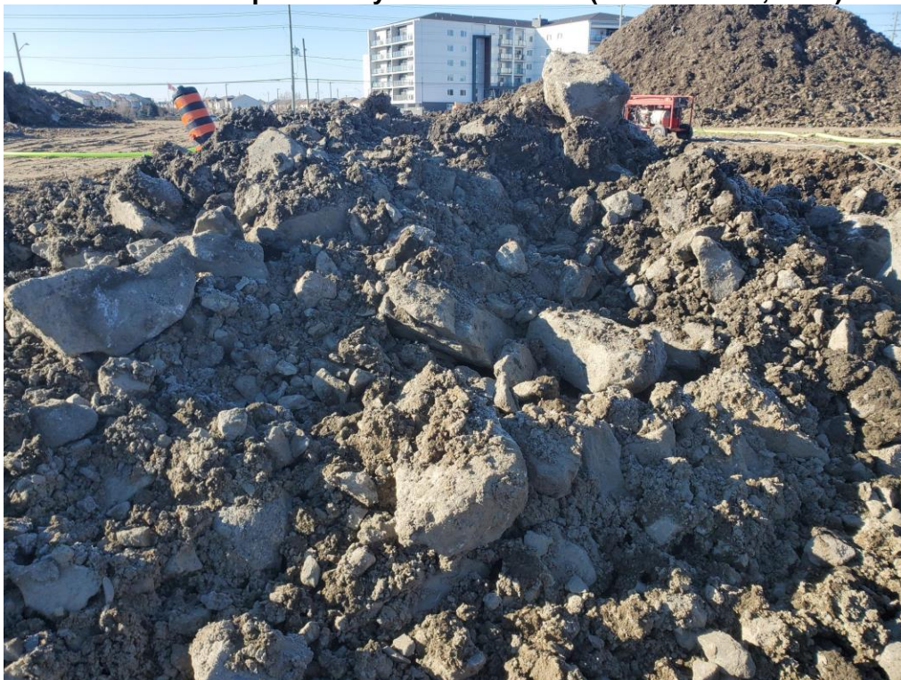
Photo 2: Stockpile of clay and boulder fill (November 24, 2021)
