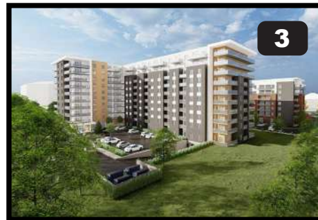
Lib Kanata | 150 Kanata Ave. (Pre-Construction, 11-ST, Mid-Rise)
