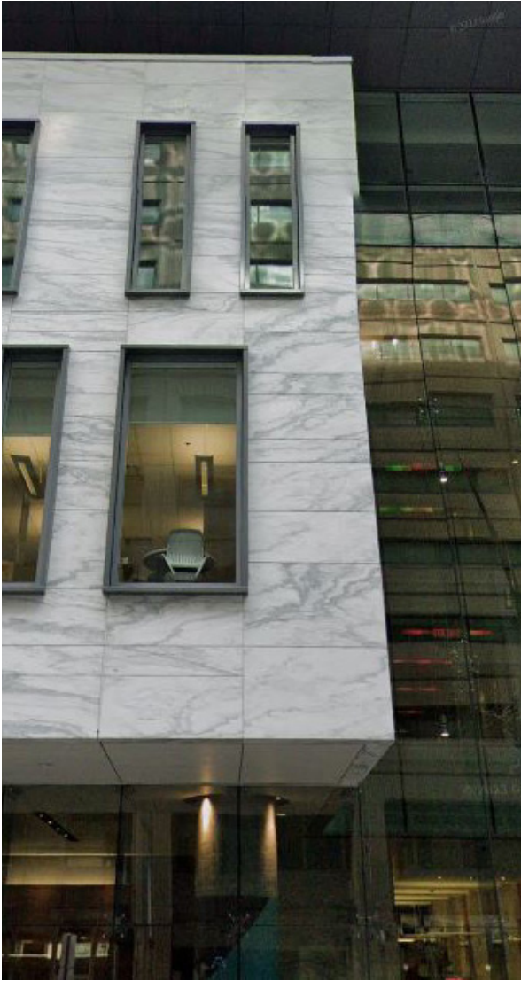
Masonry volume bisected by curtain wall
