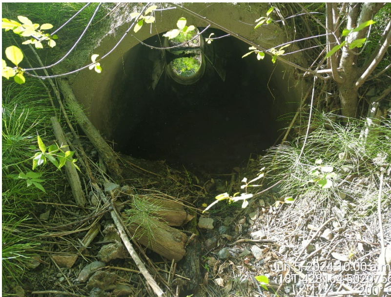
Photo 2: Culvert under the Railroad (June 5, 2024)
