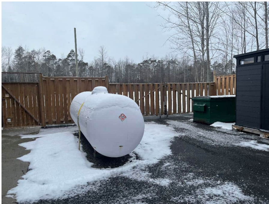
Photo 16: Large propane tank located to the north of the main building. No noted secondary containment.
