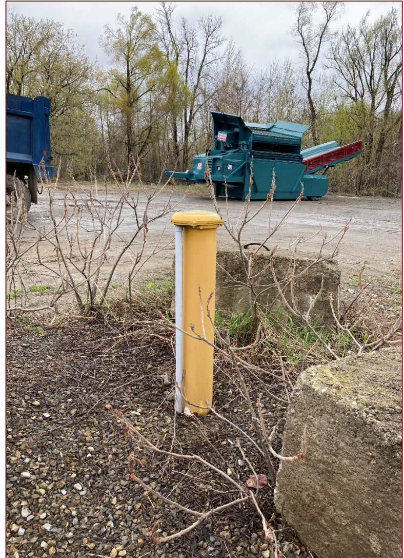
Photograph 32: Domestic water supply well for the main building.
