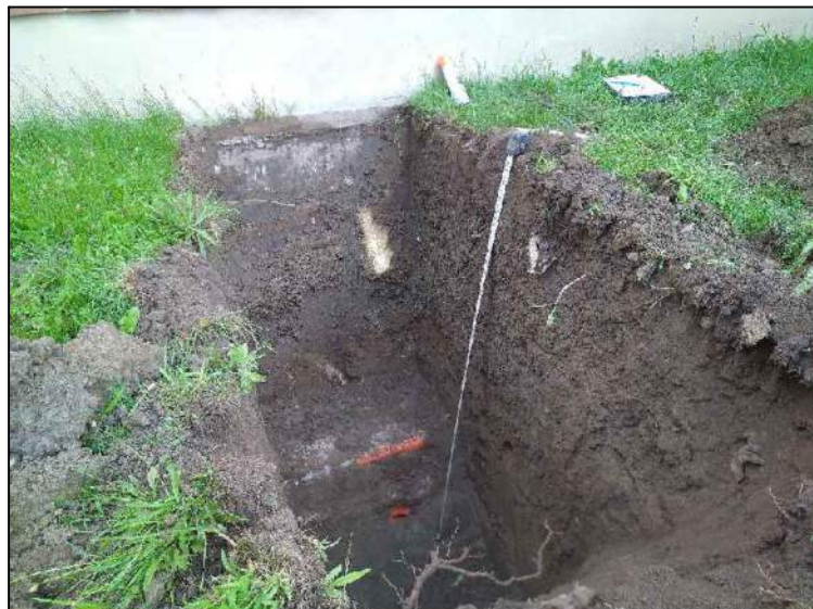
TEST PIT TP24-1 PHOTOGRAPH
