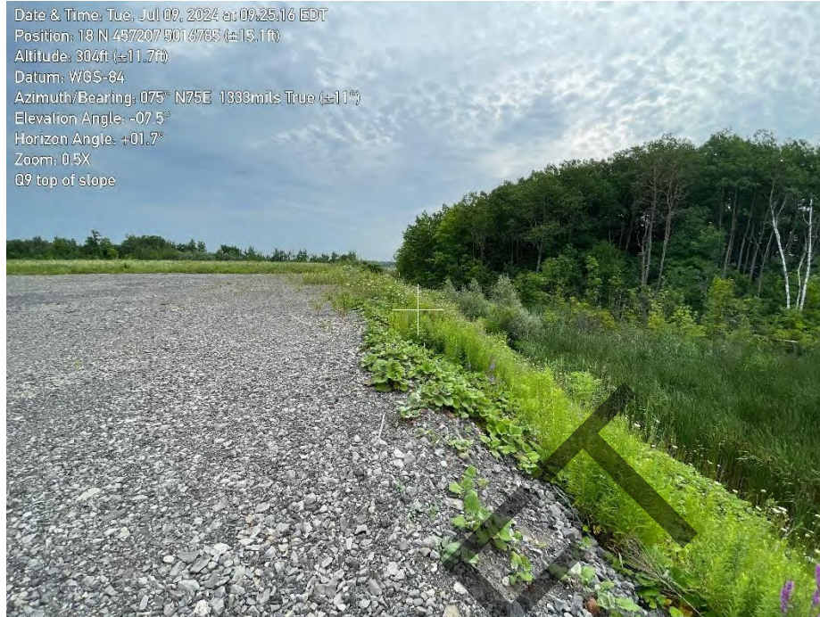
Figure 4 Top of slope, looking east
