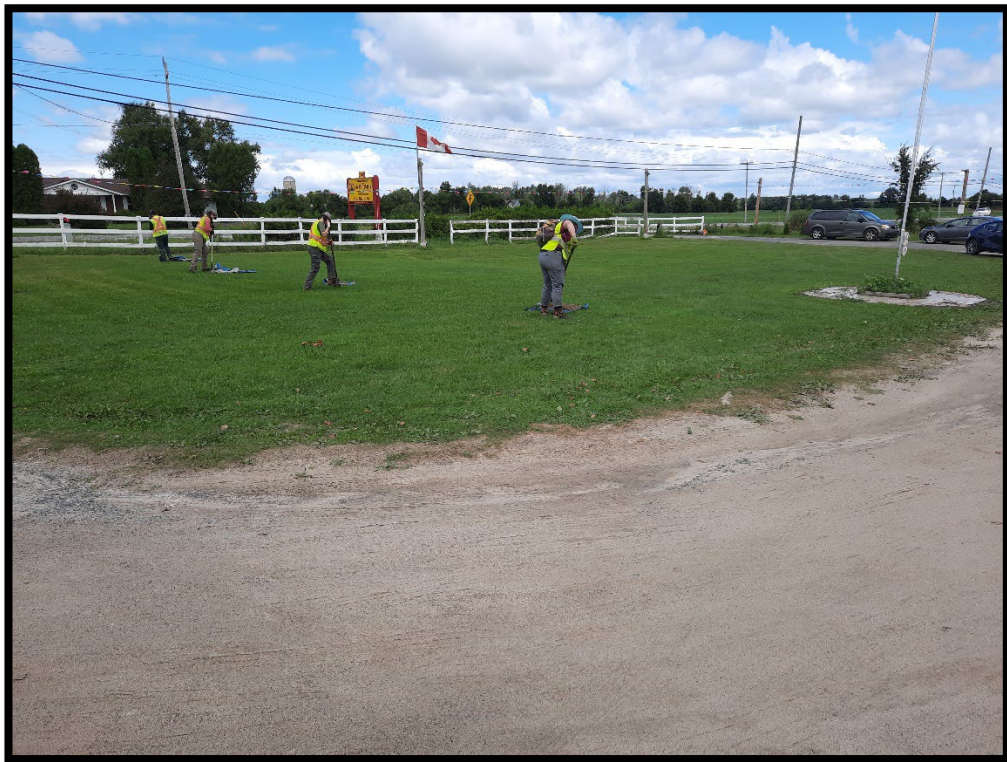
Figure 8: Test pitting in progress, (MH1289-D031).
