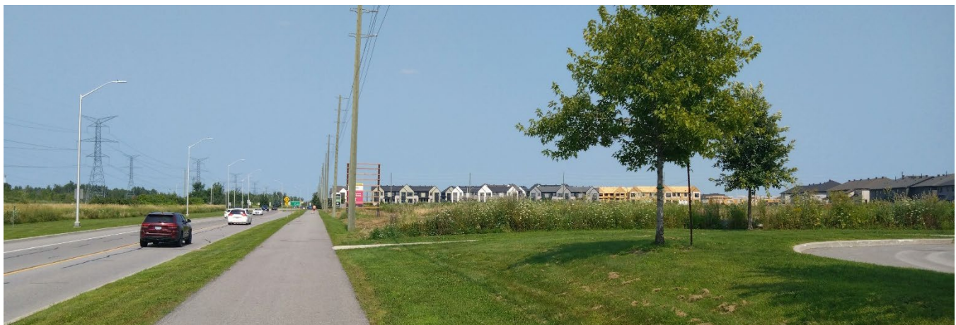
Figure 3: Brian Coburn Boulevard, forming the northern edge of the subject site. (July 2024, Fotenn)
