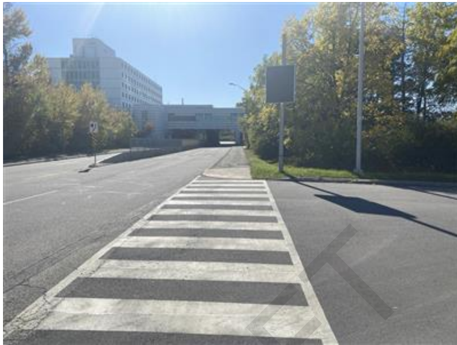
Image 9: Bus lane and infrastructure along east limit of north Study Area. Facing north.
