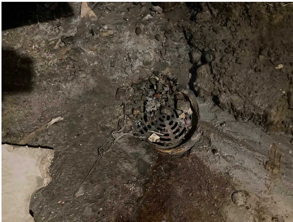
Photo 9: View of a drain in poor condition, located in the basement.
