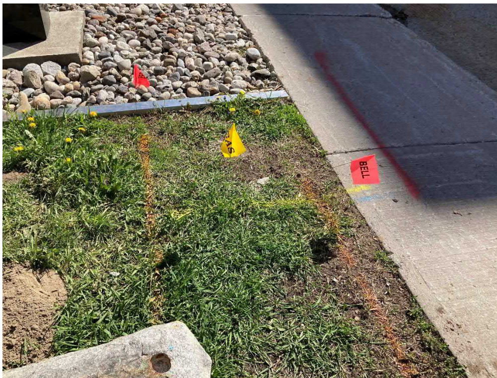
Photo 3: View of flags and spray paint markings used to identify Bell, gas, and hydro underground services.
