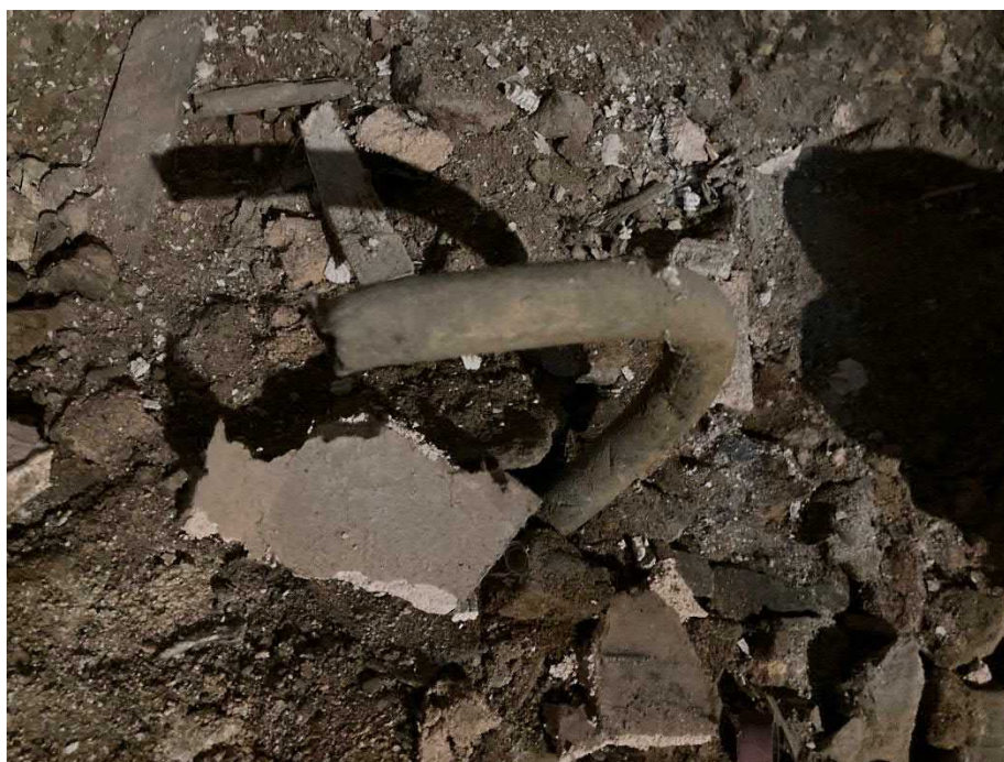
Photo 10: View of a potential lead pipe located in the basement.
