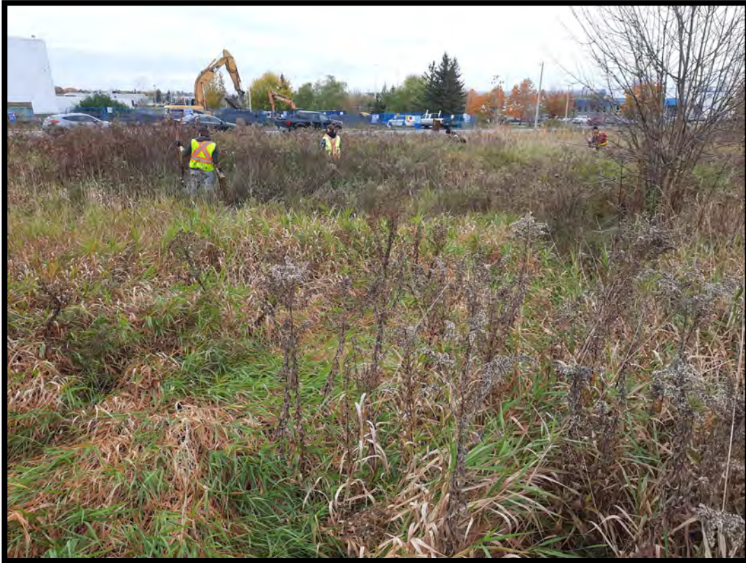
Figure 25: Test pitting in progress (D029.)
