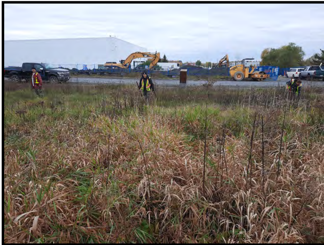
Figure 24: Test pitting in progress (D019).
