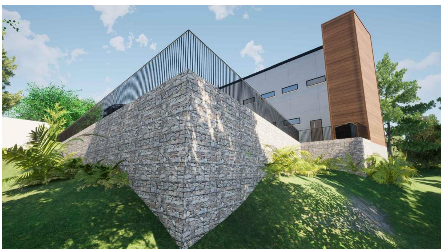
10 VIEW OF PARKING LOT GABION WALL
