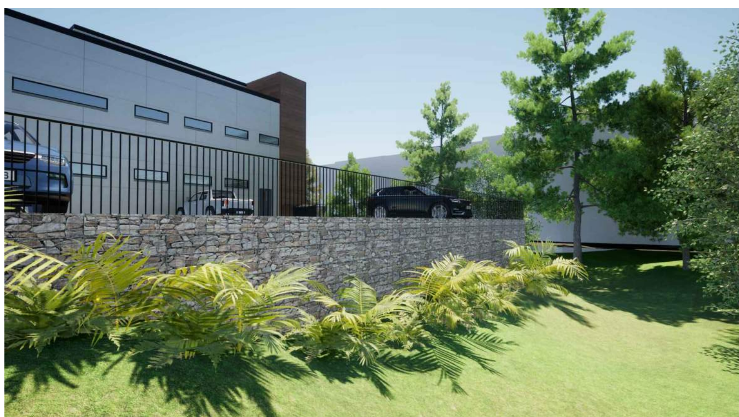
9 VIEW OF PARKING LOT GABION WALL
