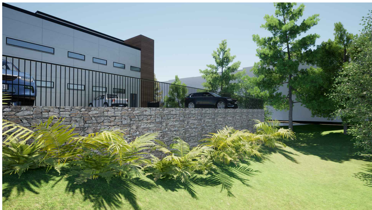
9 VIEW OF PARKING LOT GABION WALL
