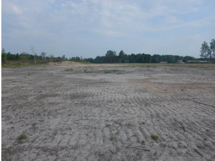
Photo 1: Cleared Area (June 2, 2023).
