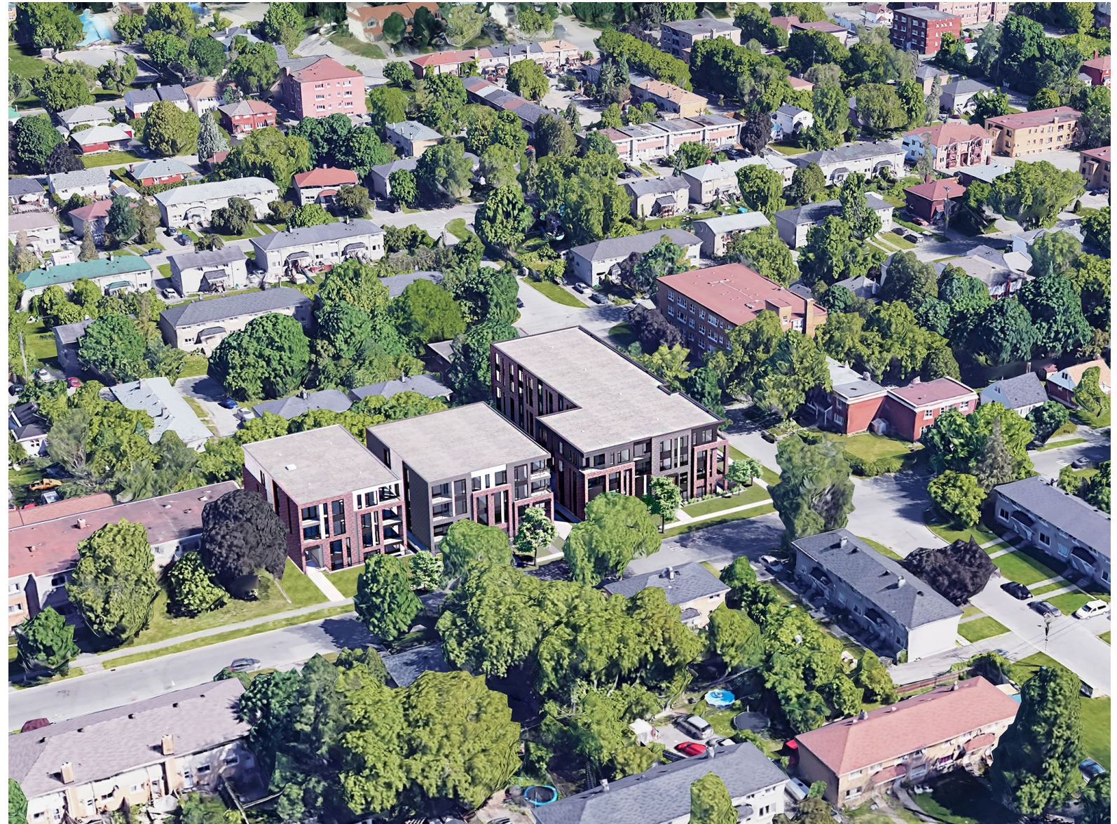
View Looking North
