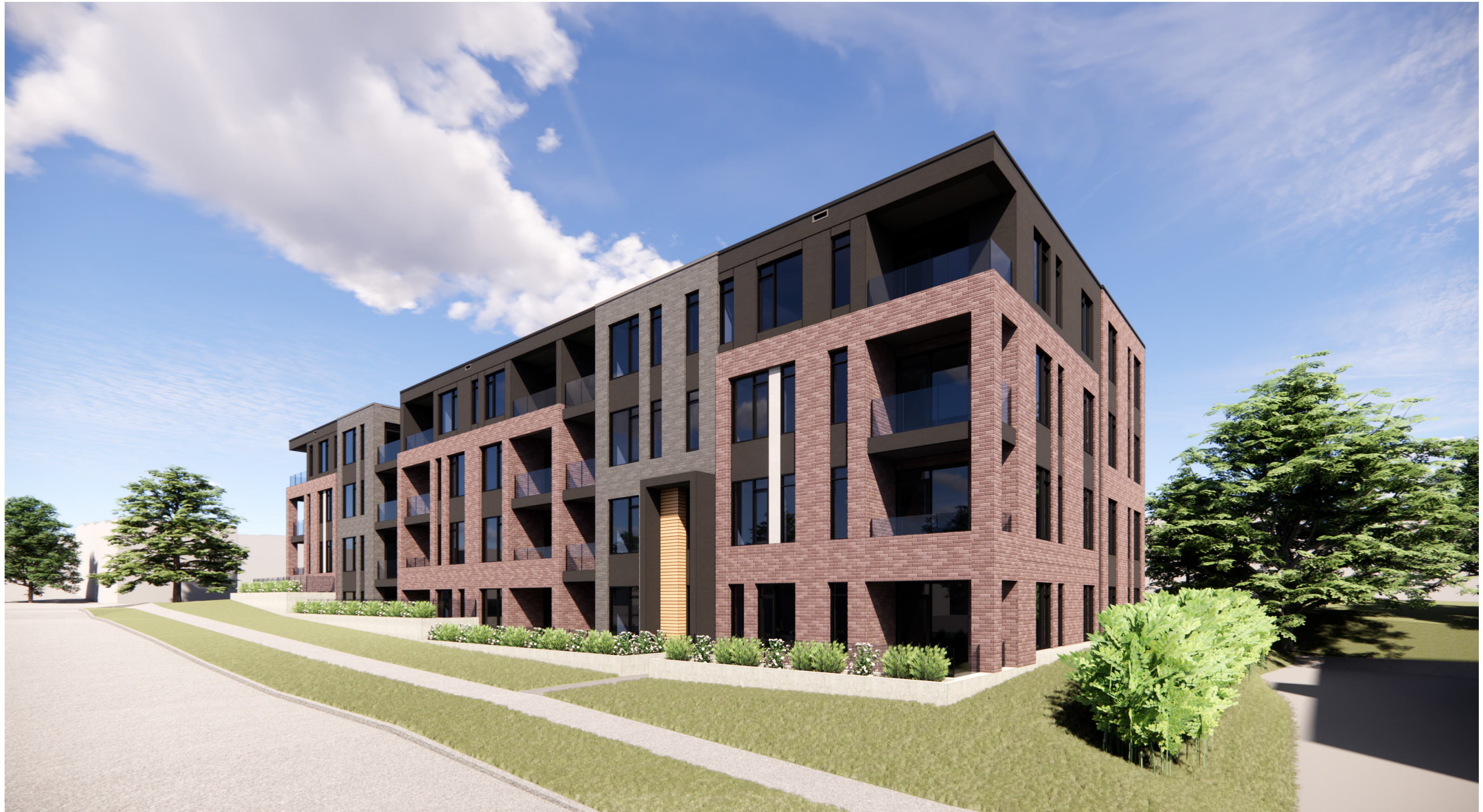
1066 SILVER STREET | VIEW FROM SILVER STREET FACING SOUTH
