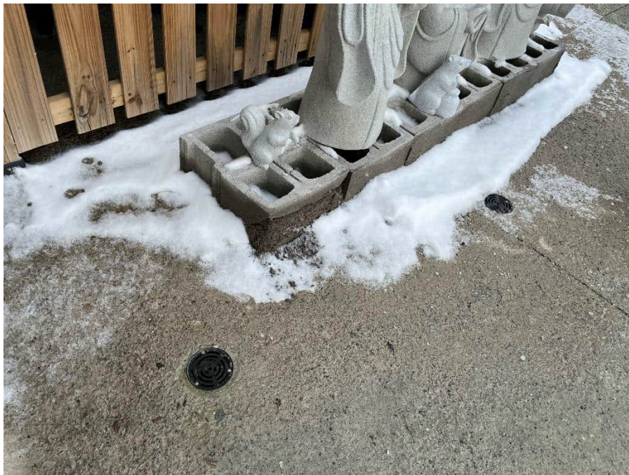
Photo 19: Exterior drains, northeast of main building.
