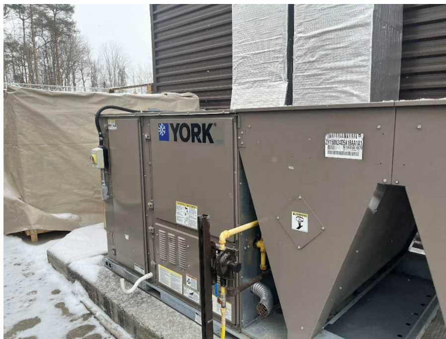
Photo 15: Forced-air furnace which supplies hot and cold air to the main building. Located to the north exterior of the Site with a concrete pad underneath.
