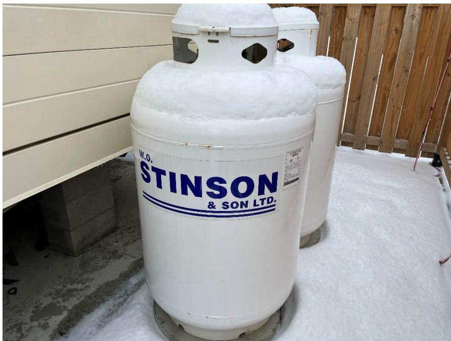
Photo 20: Two medium propane tanks which supply the kitchen trailer.
