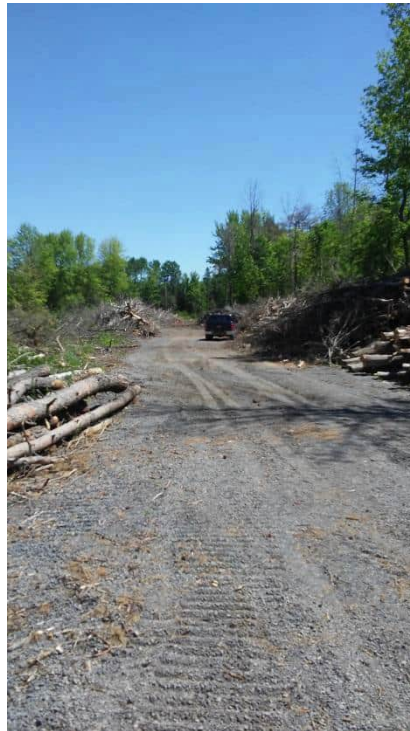
Photo 2: On-site construction laneway, view from Franktown Road
