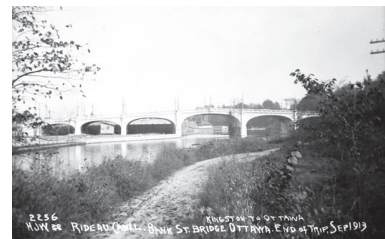
1913 photograph of south bank of Rideau Canal looking towards Bank Street Bridge (Library and Archives Canada).
