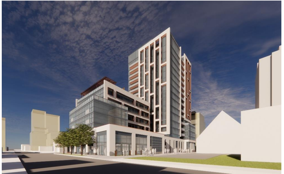
49 Looking northeast towards the proposed development along Hamilton Ave N. and proposed vehicular laneway. DIALOG.
