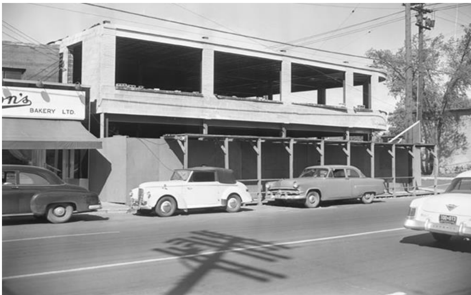
26 1191 Wellington St W, across street from site (now World of Maps), under construction. Kitchissippi Times .
