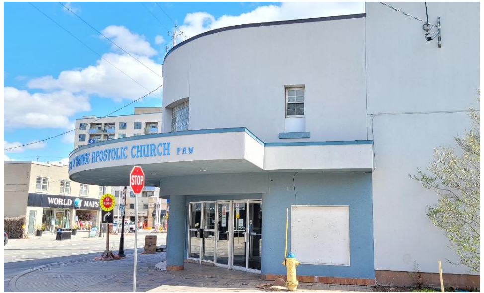
2 Cornerstone House of Refuge Apostolic Church, former Elmdale Theatre, corner of Wellington St W and Hamilton Avenue North. MTBA.
