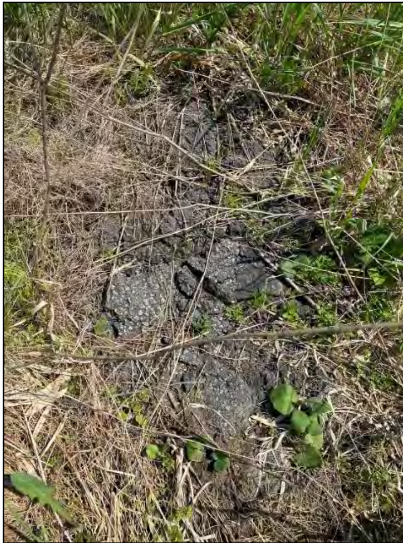
Photograph 6: View of asphalt debris at the south end of the subject property.
