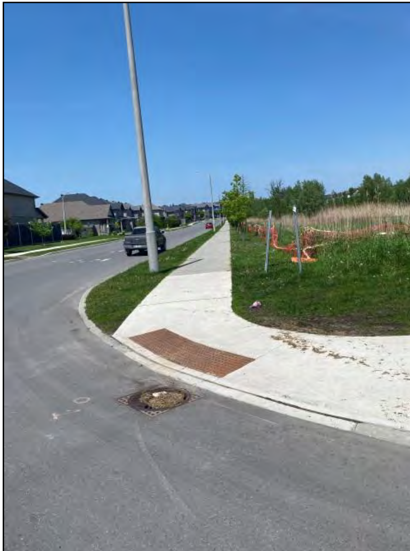
Photograph 12: Looking north along the west property boundary and Spring Valley Drive. A stormwater catch basin is in view at the north-east corner of Joshua Street and Spring Valley Drive.
