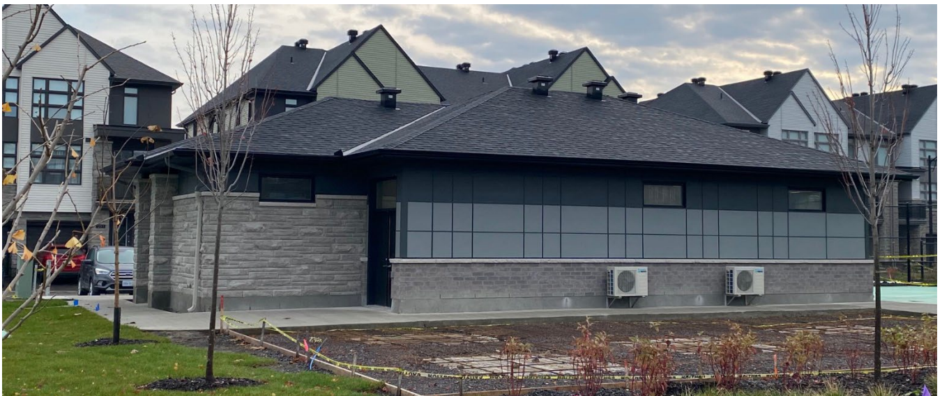
Figure 9: Elevation of the accessory building for garbage facilities and bike storage at Casey Court, similar to the proposed development.
