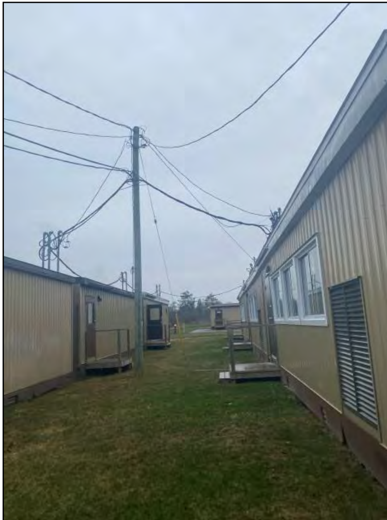
Photograph 7: View of portable classroom units and overhead electrical wires on the west side of the building.
