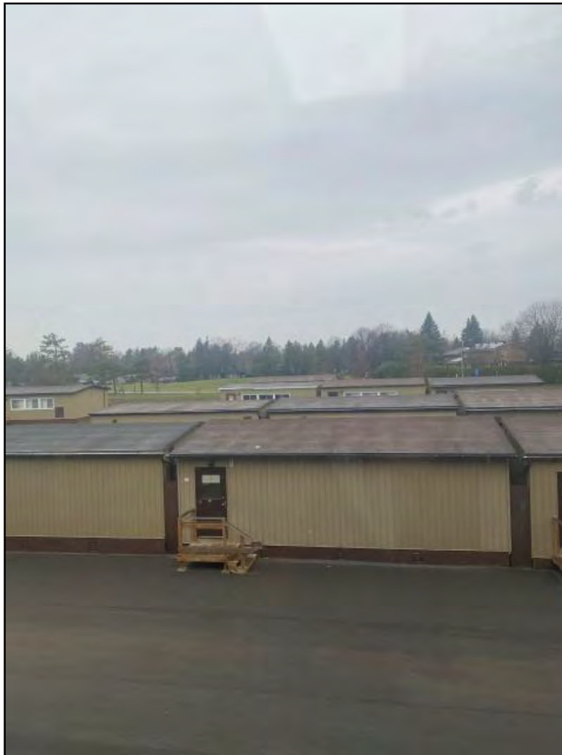
Photograph 10: Looking north-west at the proposed location of the new addition. Portable classroom units are in view.
