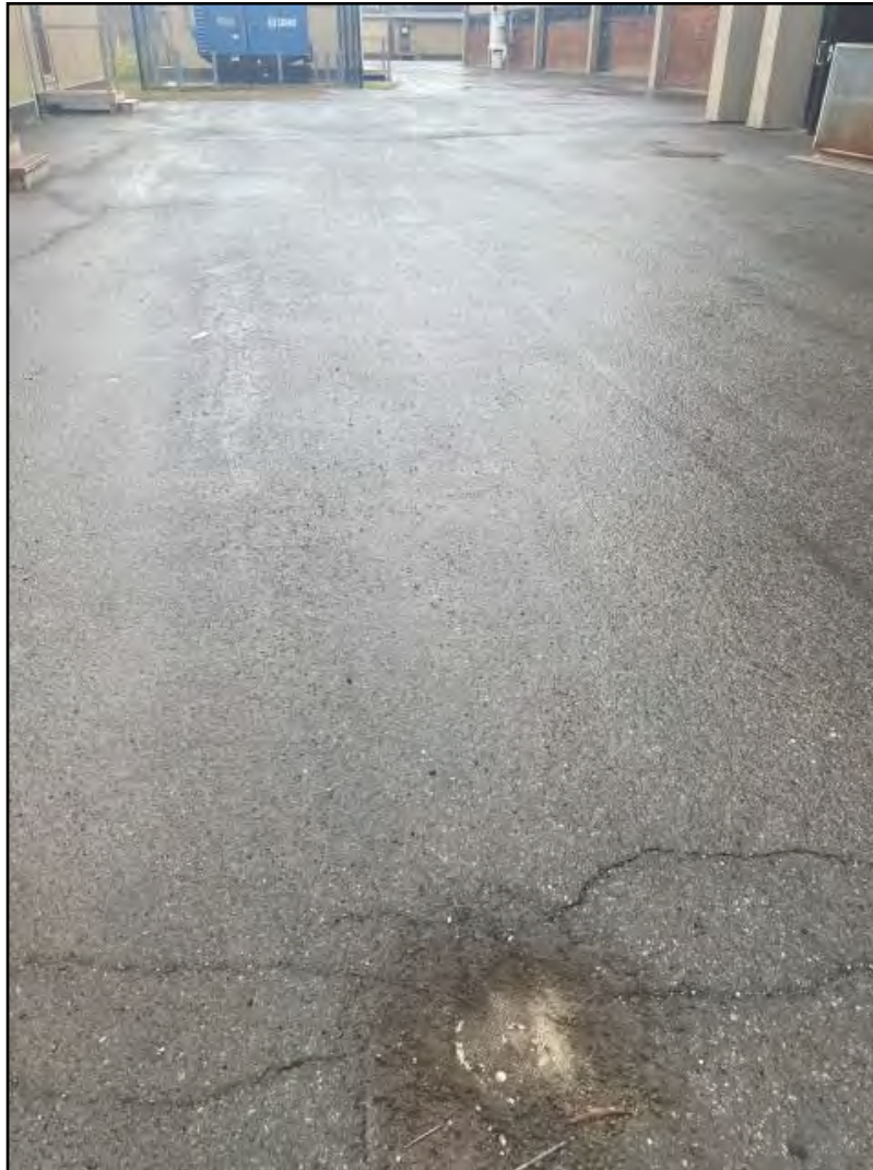
Photograph 5: View of a flush mount cover for a monitoring well on the south-west side of the building. The monitoring well is within the PHC impacted area.
