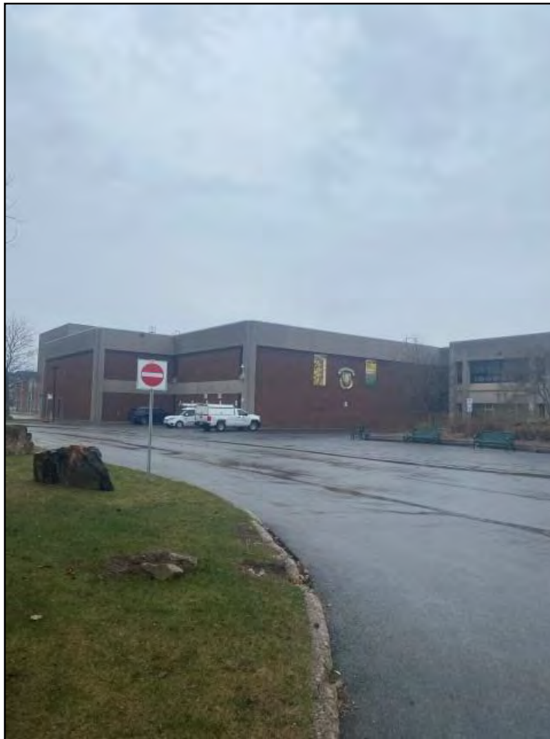
Photograph 1: Looking south at the north-east side of the building from the bus loop.
