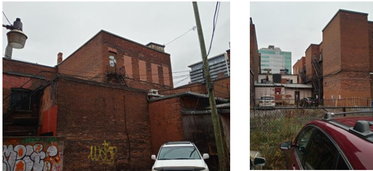
Figure 16: Views of the east façades (rear).
