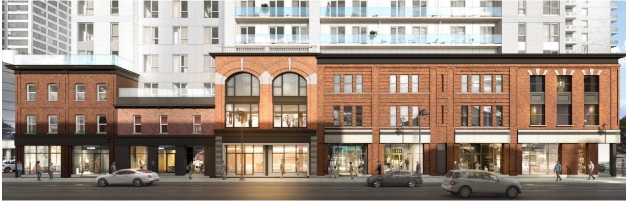
Figure 4: 115-117 As part of the Bank Street range.
