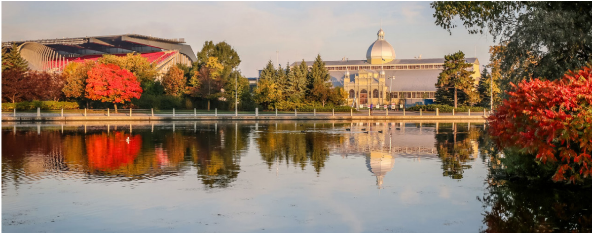
View from the Rideau Canal, from southwest of Lansdowne Park, looking northeast toward the Aberdeen Pavilion (Rideau Canal Cultural Landscape Study, Matrix Heritage, 2024 DRAFT).
