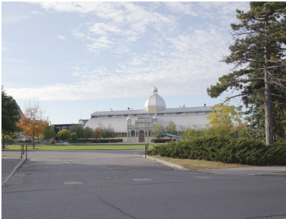
View H1.2 existing condition.
