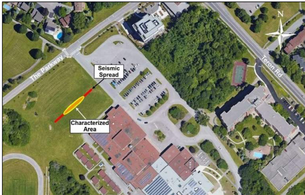
Figure 2: Location of the seismic spreads (source: Google Earth™)
