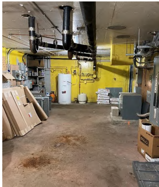
Photograph 4: View of the basement
