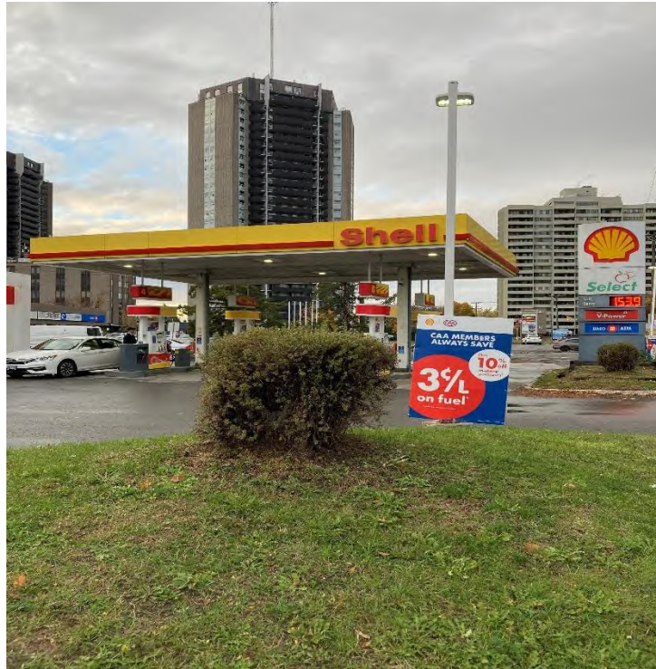
Photograph 1: View of the Phase One Property – looking north
