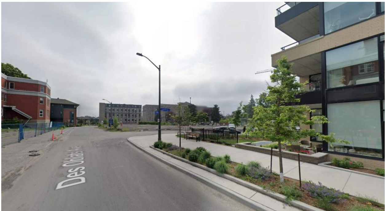
Image 4: Low to Mid-rise residential uses along Des Oblats Avenue (looking east toward Subject Property)
