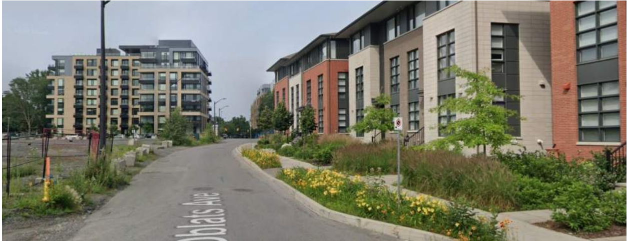
Image 1: Recently Constructed Low to mid-rise development along Des Oblats Avenue (looking west)
