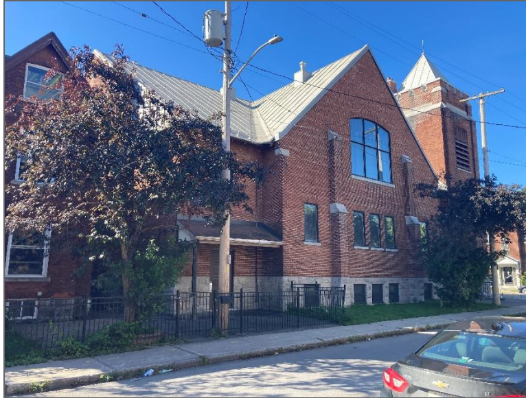
Photo 1 – Site Building (north elevation).
