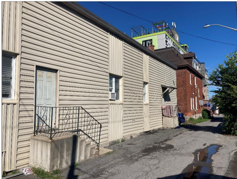
Photo 2 – Site Building (east elevation).
