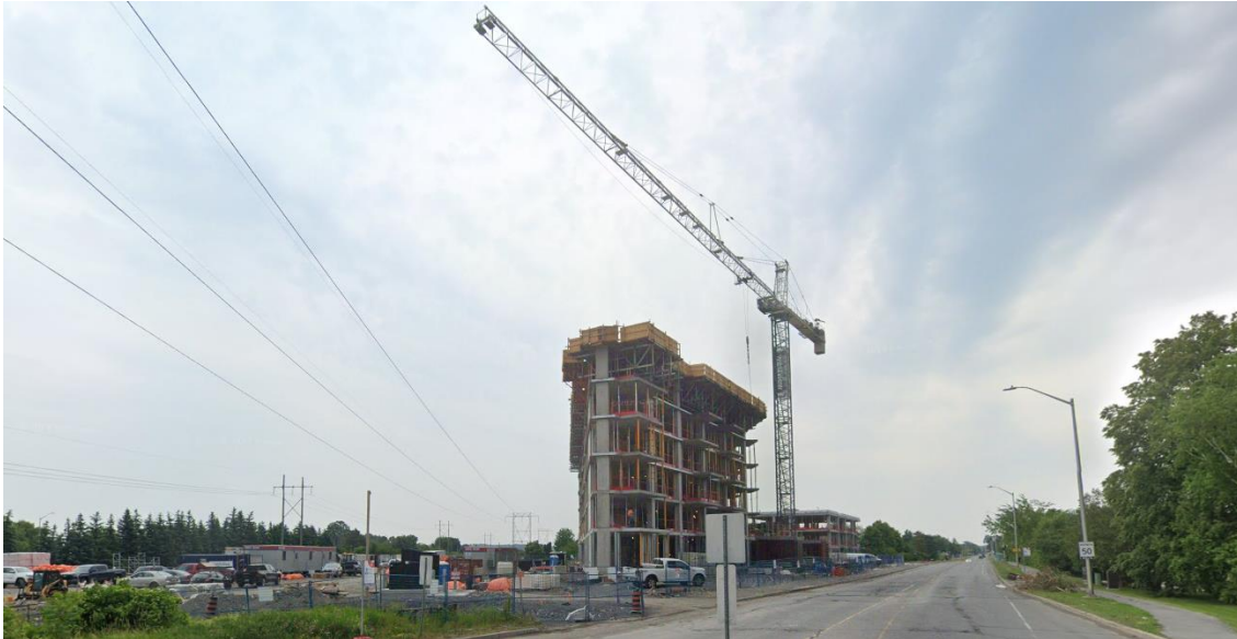
Figure 20: Development at 1151 Teron Road under construction as of June 2023.
