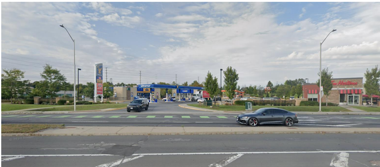
Figure 23: Existing Commercial Plaza, 401 March Road.
