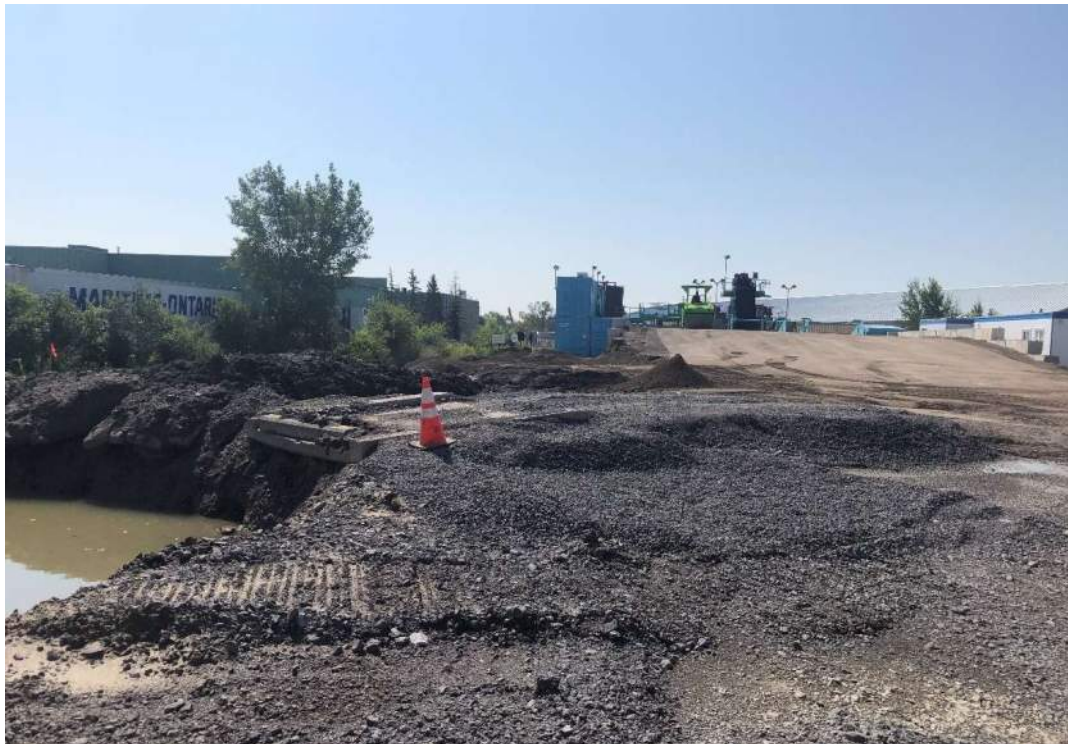
Photograph 2: View of Liquid Soils Treatment Facility
