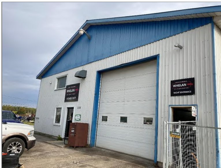
Photo 4 – Site Building (southwest elevation).
