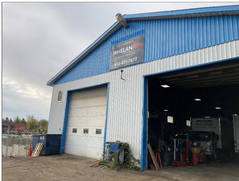
Photo 2 – Site Building (northeast elevation).
