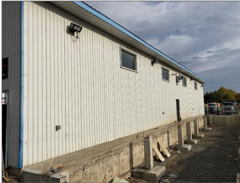
Photo 3 – Site Building (southeast elevation).
