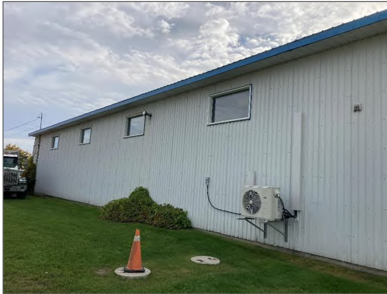
Photo 1 – Site Building (northwest elevation).
