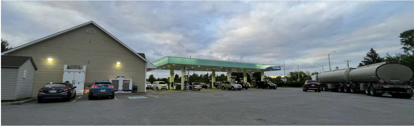
Exhibit F: Subject Property from its western side
