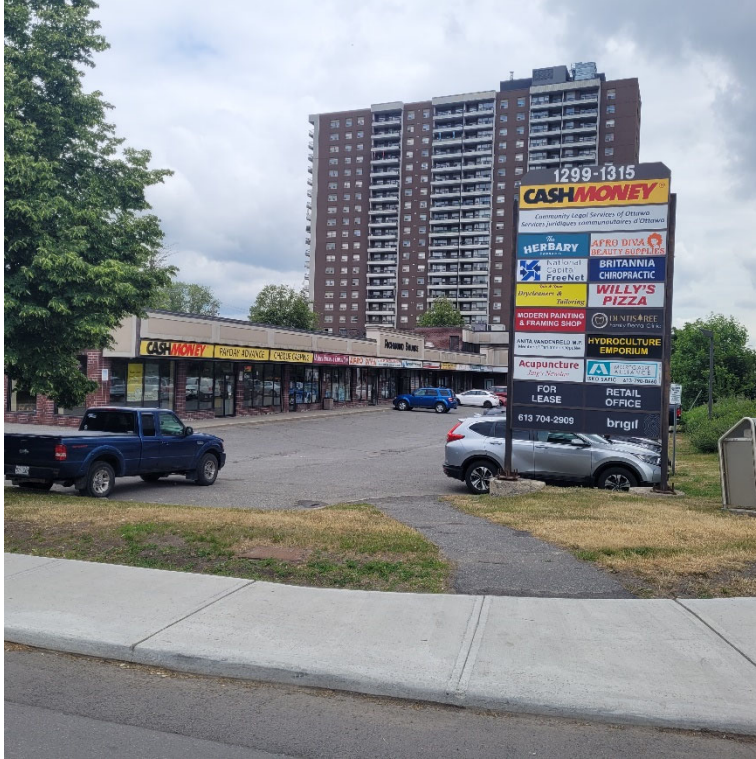
Photograph 1: View of the of the west portion of the Phase One Property looking northeast. View shows the 1-storey plaza building on the central and west portion of the Property.
