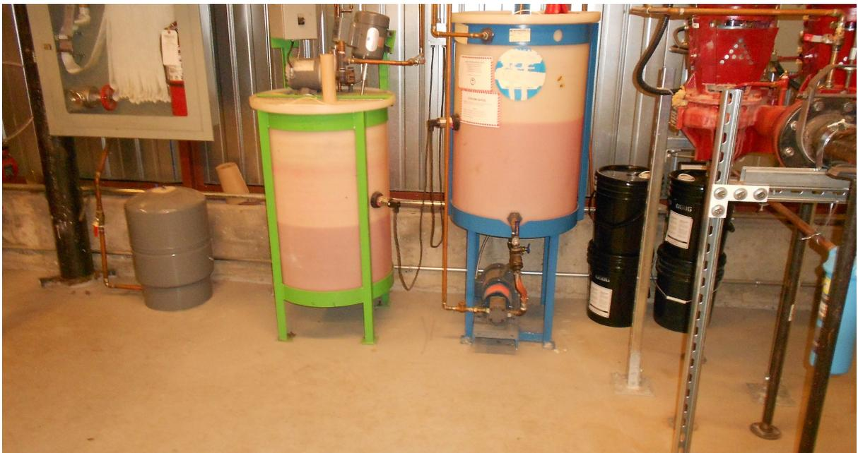
*Photo 24 Typical penthouse glycol loop system and reservoir tanks.*
