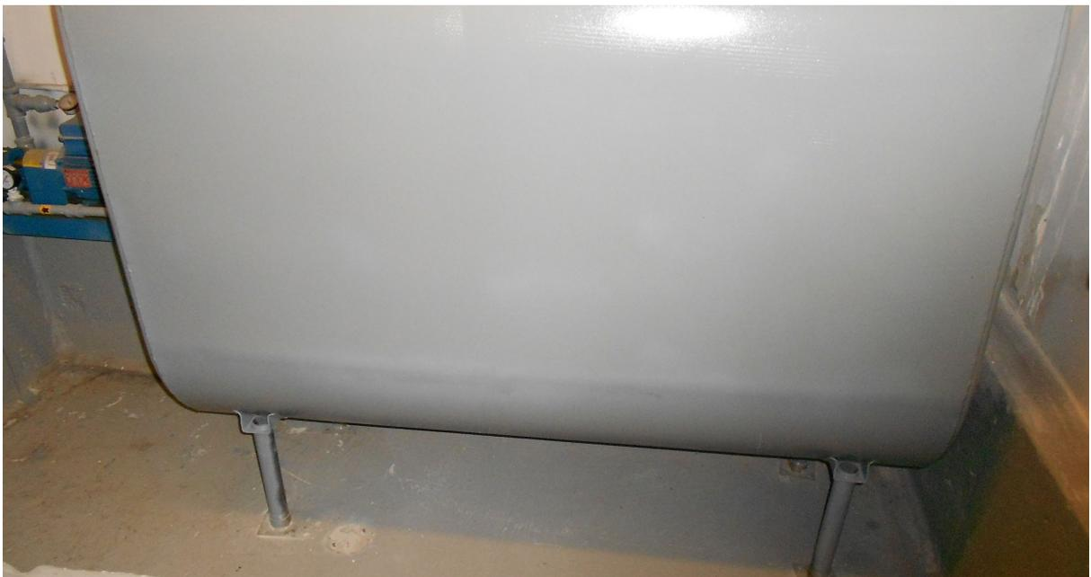
**Photo 20** *View of bulk diesel tank on ground floor of Tower 3 (feeds day tank located in Tower 3 penthouse).*
