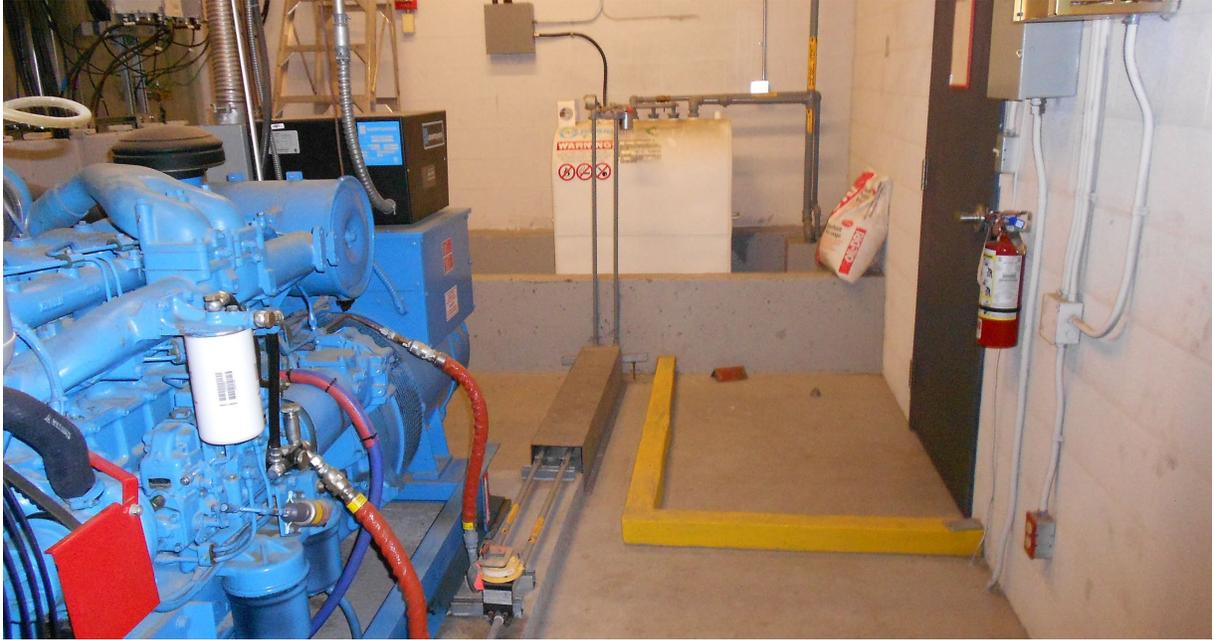
**Photo 19** *View of diesel generator and day tank located in penthouse of Tower 3.*
