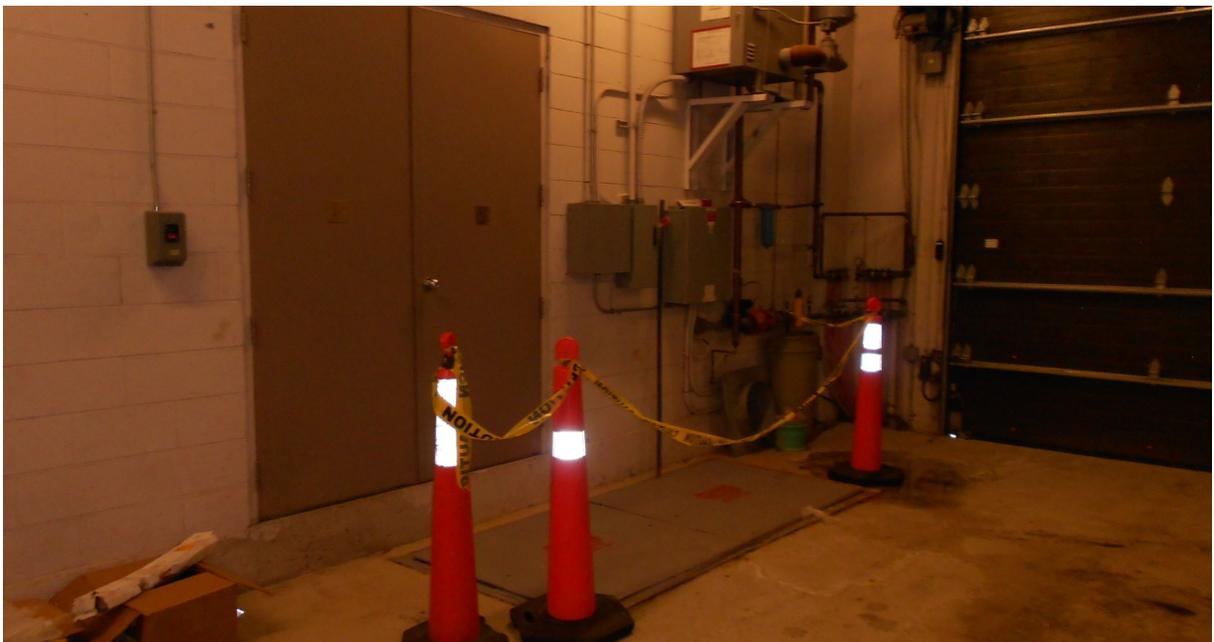
*Photo 22 View of sump pump pits and glycol system for Tower 2 basement loading ramp with trench drain.*
