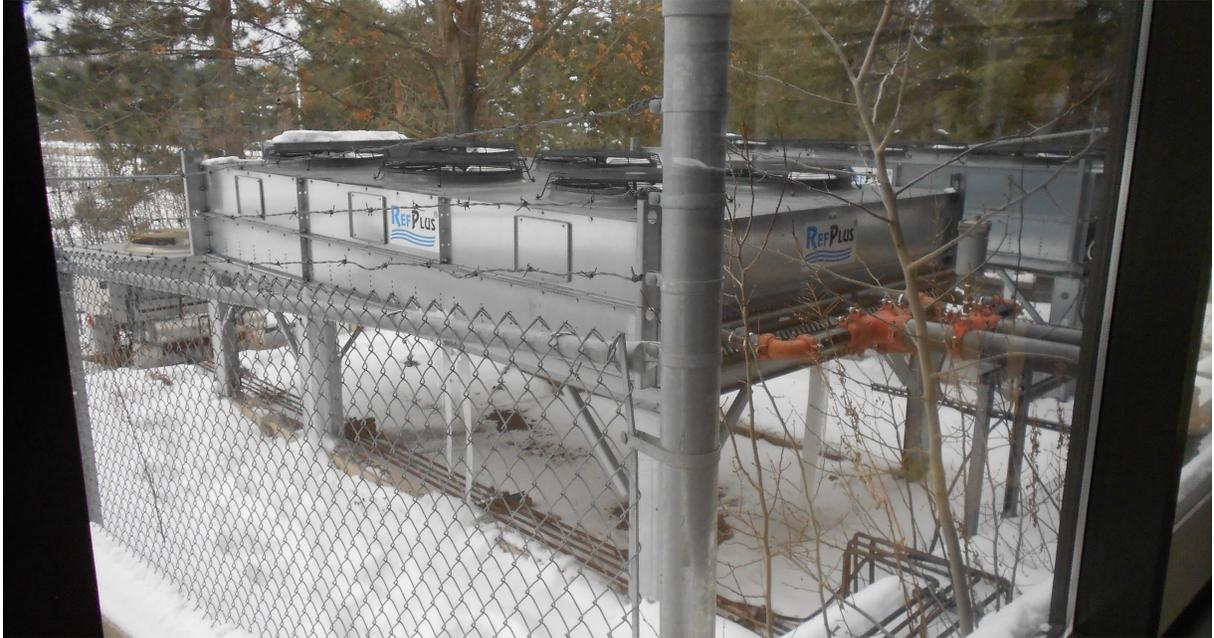
**Photo 25** Typical exterior heat exchanger system (glycol or refrigerant).
