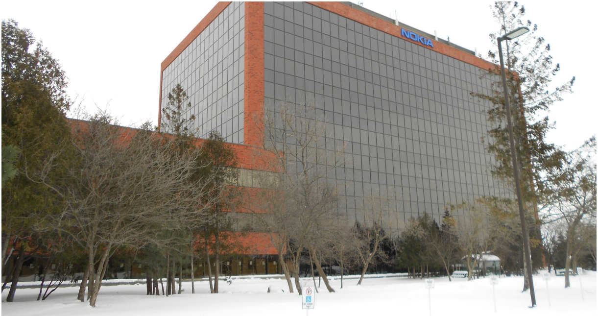
Photo 3 View of Site Building (Link 2 and Tower 3), facing east.
