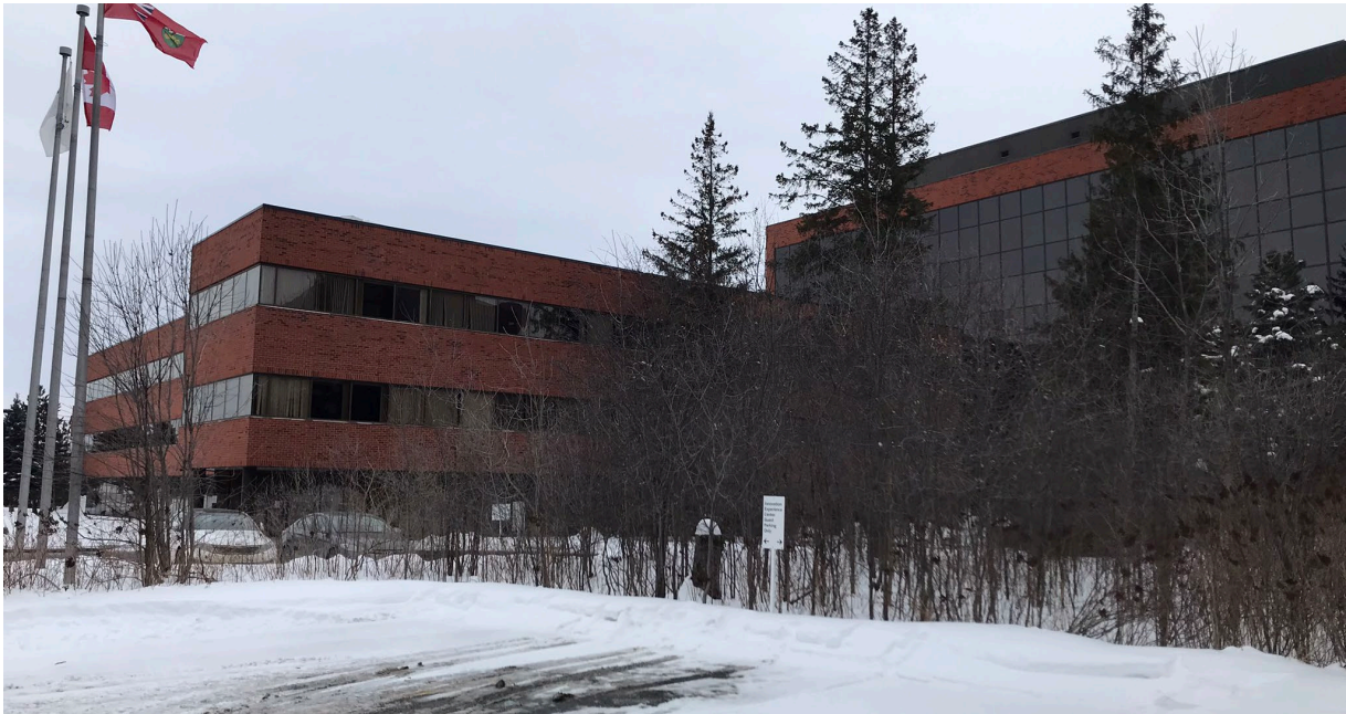
Photo 1 View of Site Buildings (Corporate Tower and Tower 1), facing north.
