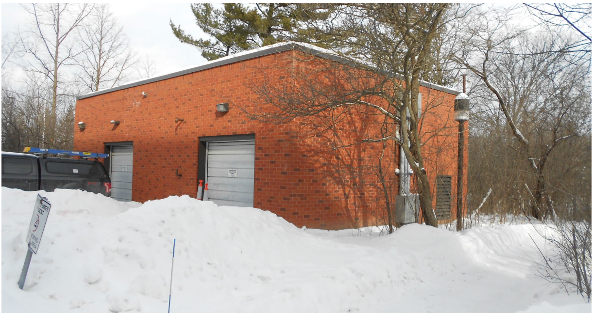
Photo 6 View of Site Building on northeast portion of Property, with Hydro Vault (left portion of building) and Diesel Generator and Tank (AST; right portion of building) on the interior, facing north.
