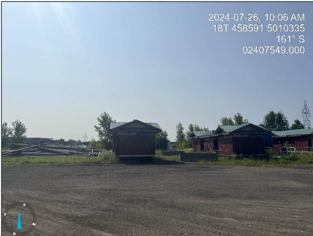
Photograph 14: Exterior Old Canal Shelter Storage Area (6622 Bank Street).
