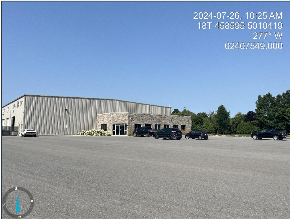
Photograph 1: Exterior view of the on-Site Building (6622 Bank Street).
