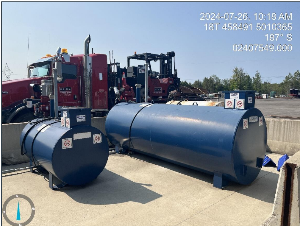
Photograph 8: Three Exterior Fuel ASTs (6622 Bank Street) - PCA 2.
