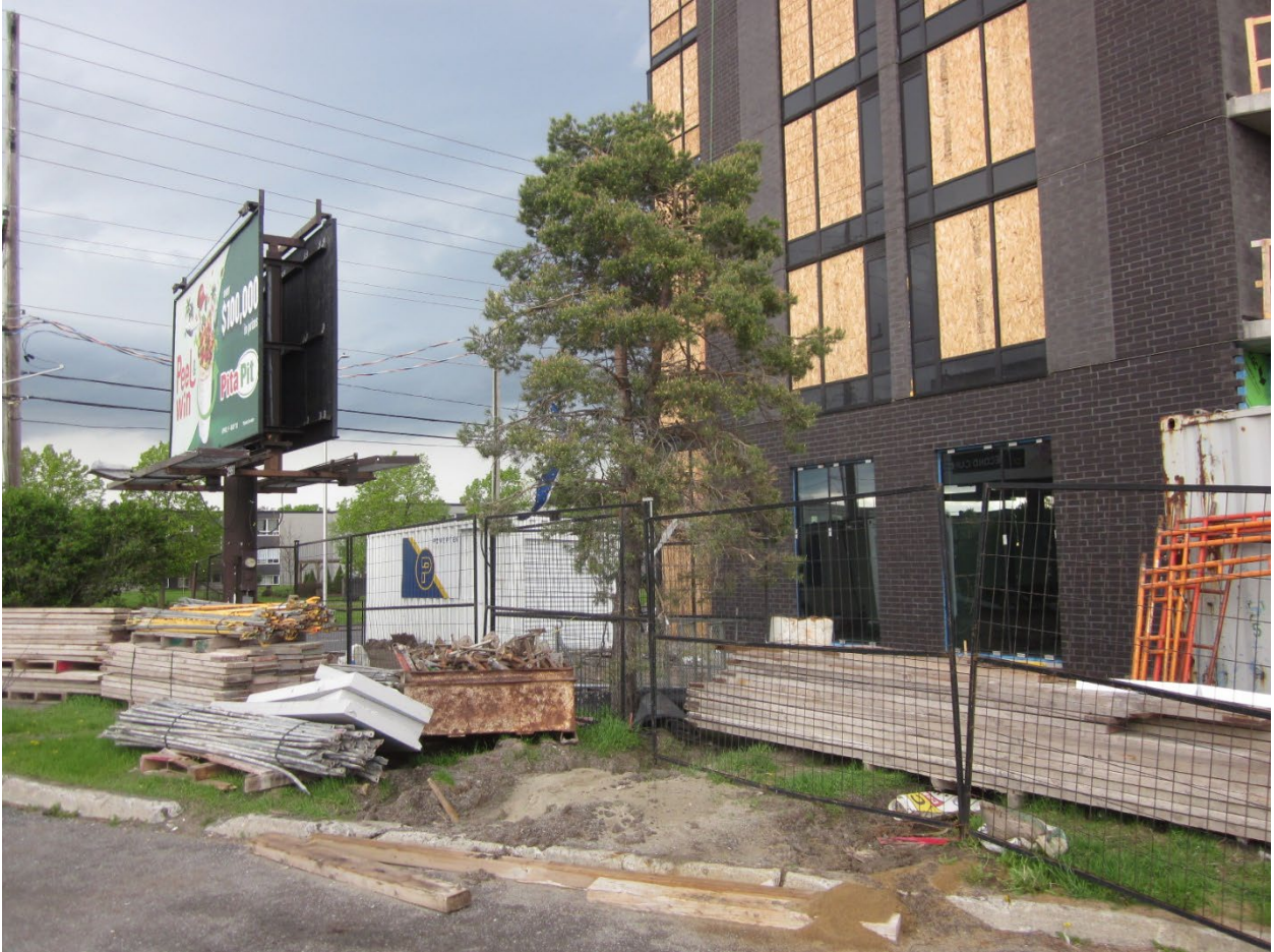
Picture 3. Current condition of tree #4 (Scots pine) at 2140 Baseline Road.
