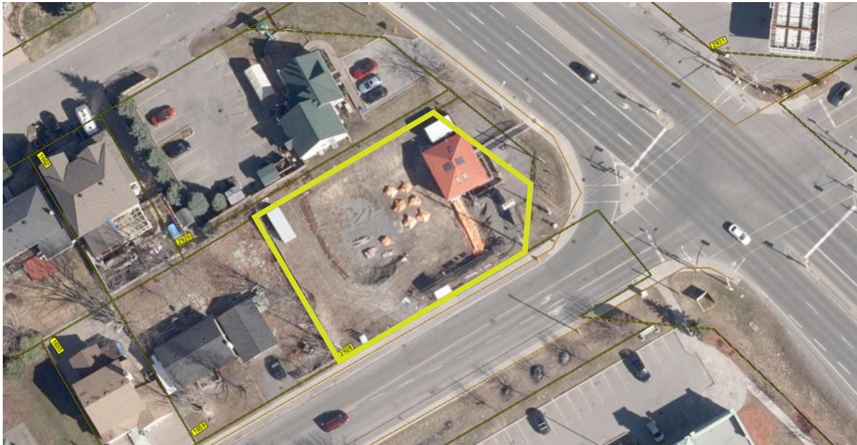
Figure 1: Aerial of Subject Site (Source: GeoOttawa)
